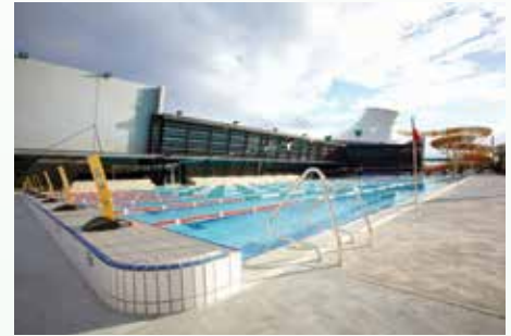
The new $45 million Glen Eira Sports and Aquatic Centre boasts a state-of-the-art pool water filtration system, thanks to Waterco.
