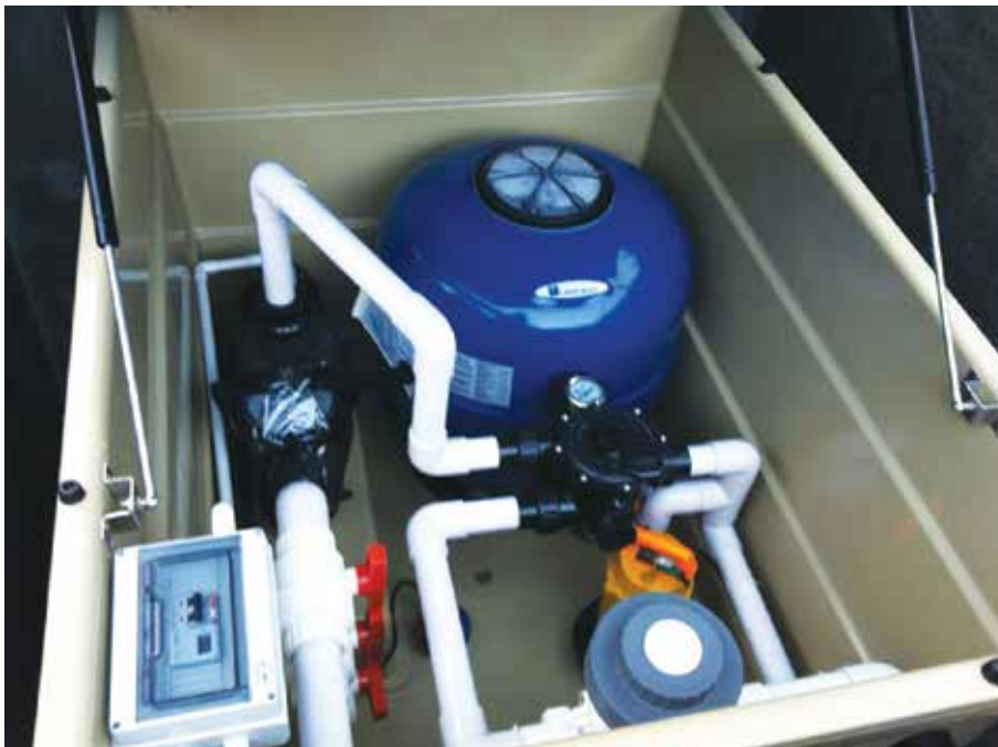
◀ WG600 all-in-one machines were customized specially for this development, the filter enclosures include a pump, filter and controller.
