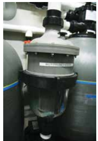
MultiCyclone filters up to 80% of the pool's dirt load before it reaches the pool filter.
