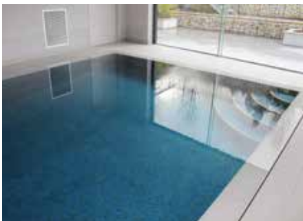
50m 3 indoor, in ground fully tiled concrete pool with an overflow wet edge.
