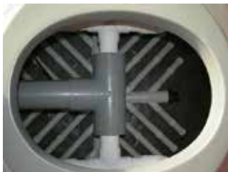
Lateral under drain system
